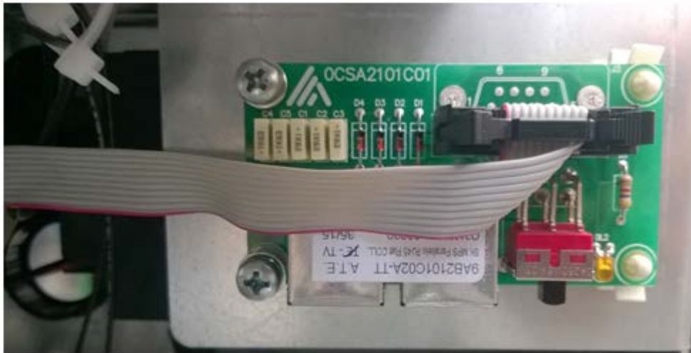
Figure 30 – Parallel Card Flat Cable Installation
